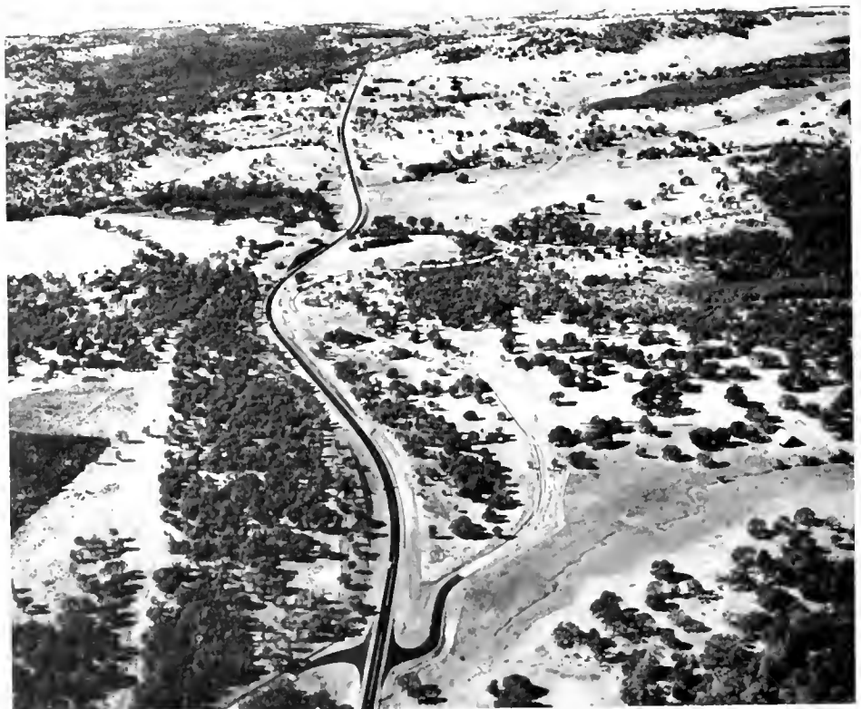
Aerial photo showing realigned US 50 from 2.25 miles east of Clarksville to Shingle Springs. Old route shown with dotted line on right.
